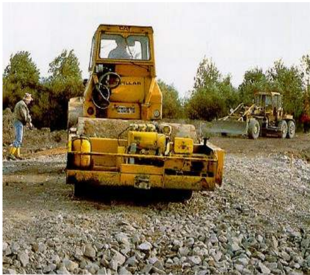
Linköping uses synthetic gravel made from PFBC ashes
